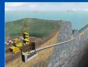
Micro-tunnel Shore Crossing
