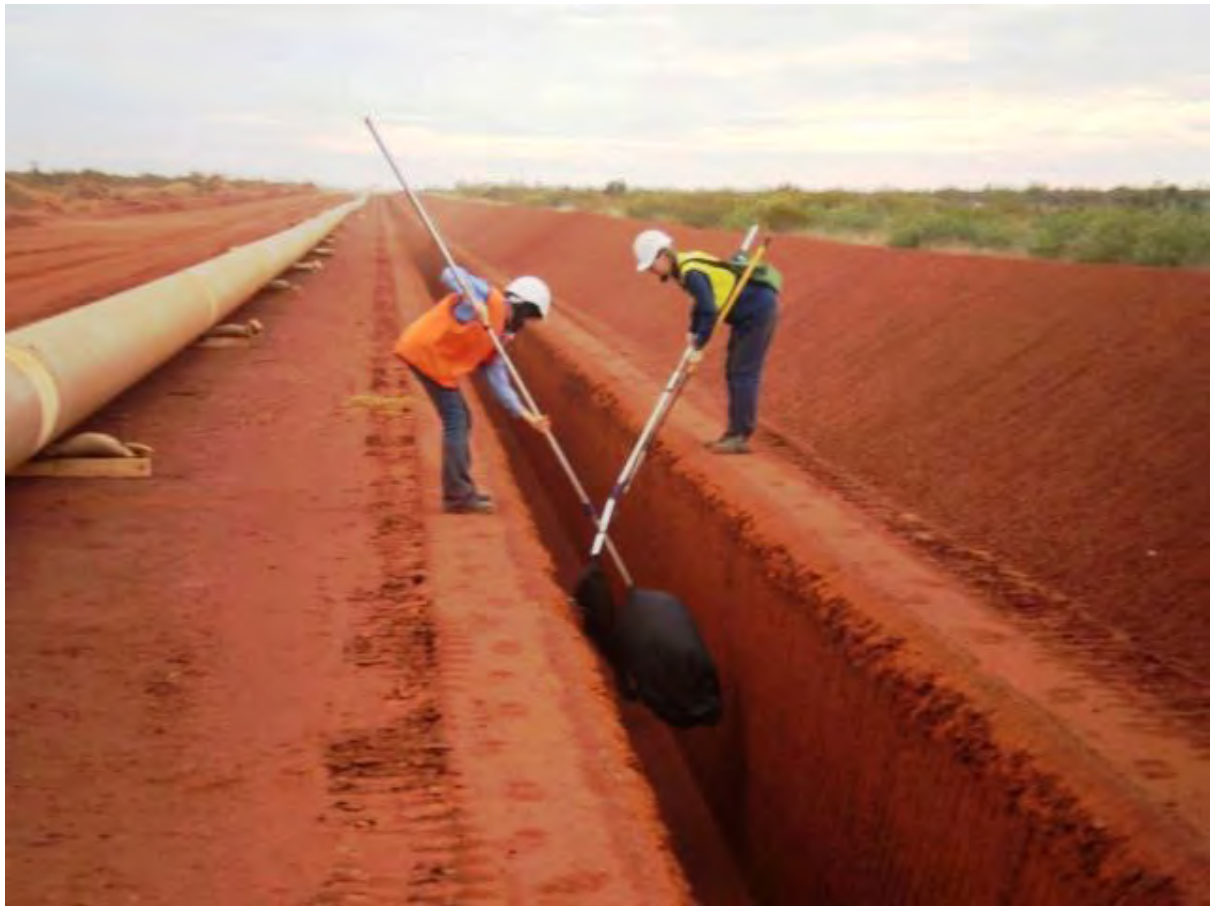
Figure 2.1: Fauna Handlers Clearing a Pipeline Trench
