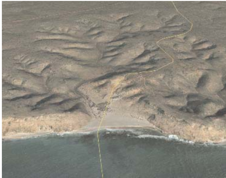
Fig 3.2 Aerial viewing east towards Flacourt Bay showing proposed pipeline corridor and existing road terminating on ridgeline south of beach.
