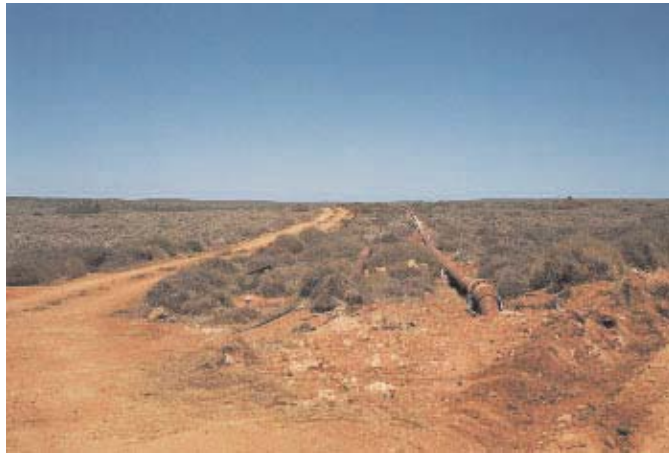
Figure 2.10 - View westerly from terminal tanks towards the central uplands showing main oil distributor pipe. Views along the pipe easement are in contrast to views adjacent the pipeline easement where low vegetation can screen pipeline views.
