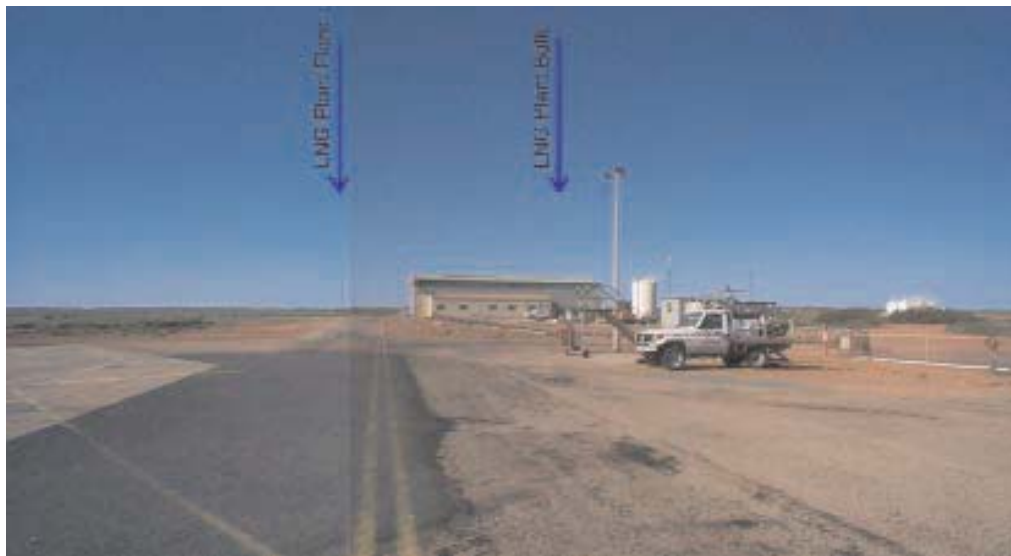
Figure 3.17 – This view is looking north north-east from the New Airport passenger terminal at Barrow Island 9.7km south west of the of the Proposed LNG Plant site.
