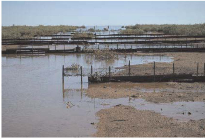
Figure 2.13 - View west showing existing pipeline easement through the shoreline vegetation and rehabilitation works involved with mangrove re-establishment.
