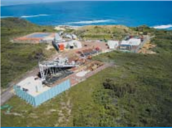
Plate 6-2: Horizontal Directional Drilling Operation
