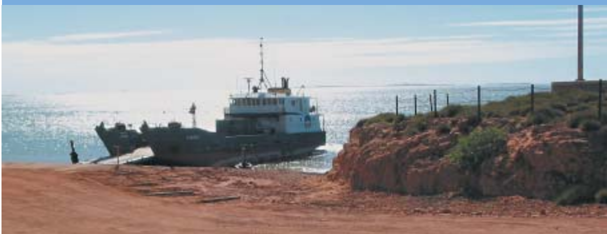
Plate 6-11: Existing Barge Landing
