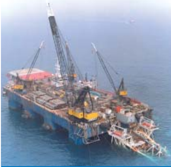
Plate 6-10: Typical Pipe-lay Barge
